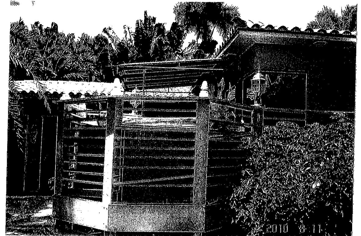
EXISTING EAST SIDE OPEN WOOD PORCH
