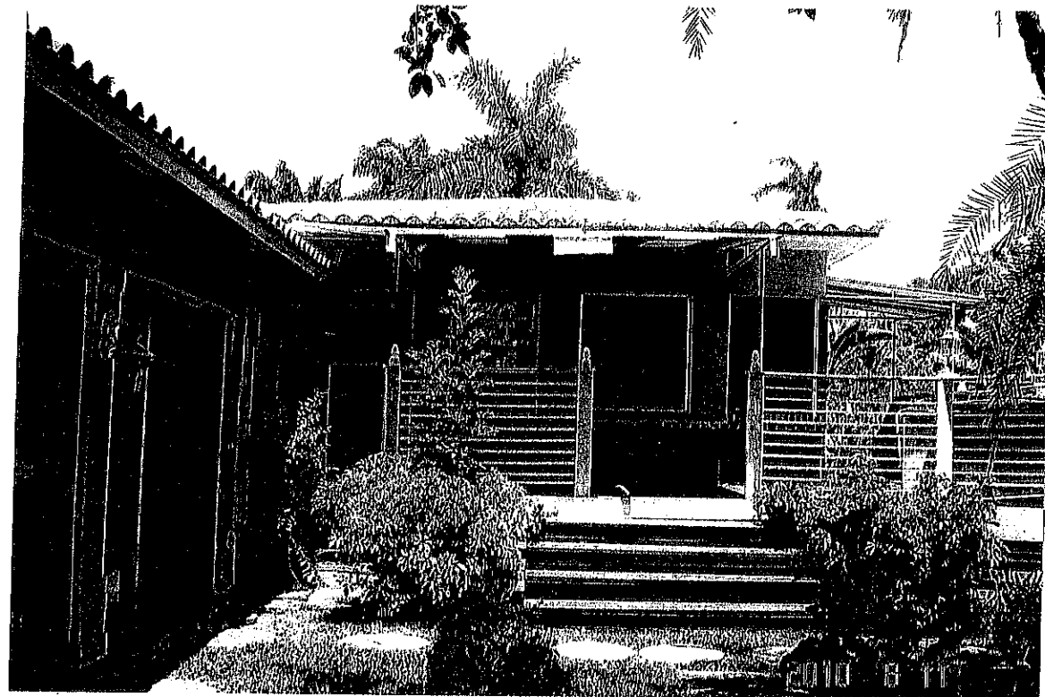
EXISTING SOUTH EAST CORNER PART OF THE HOUSE
