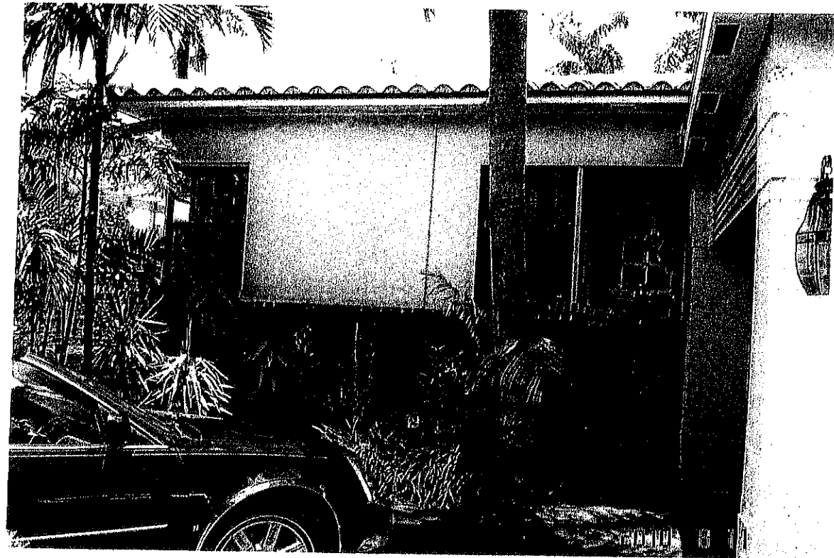
EXISTING NORTH ELEVATION - ENTRANCE OF THE HOUSE
