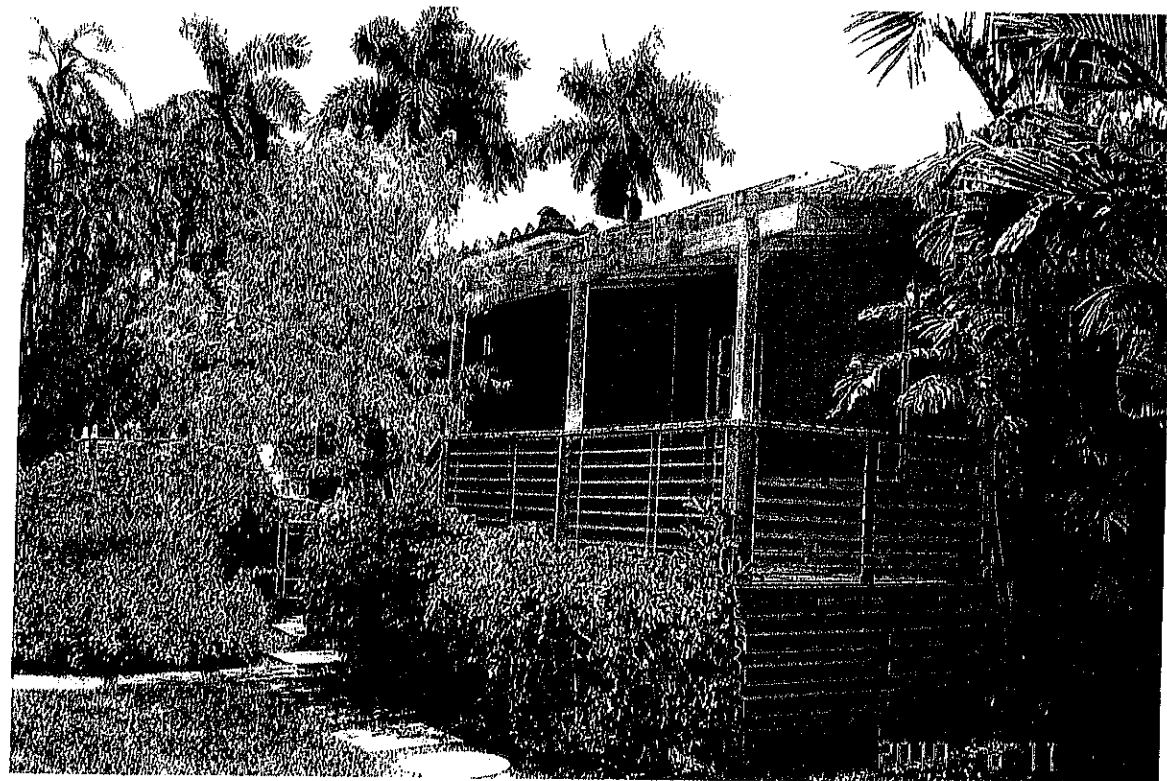
EXISTING NORTH-EAST SIDE CORNER
